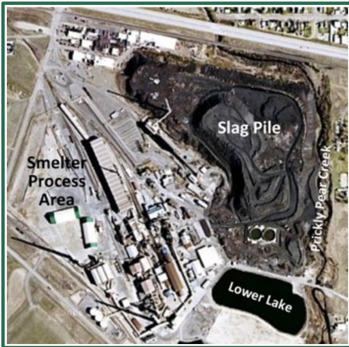
Aerial view of former ASARCO Smelter before cleanup
