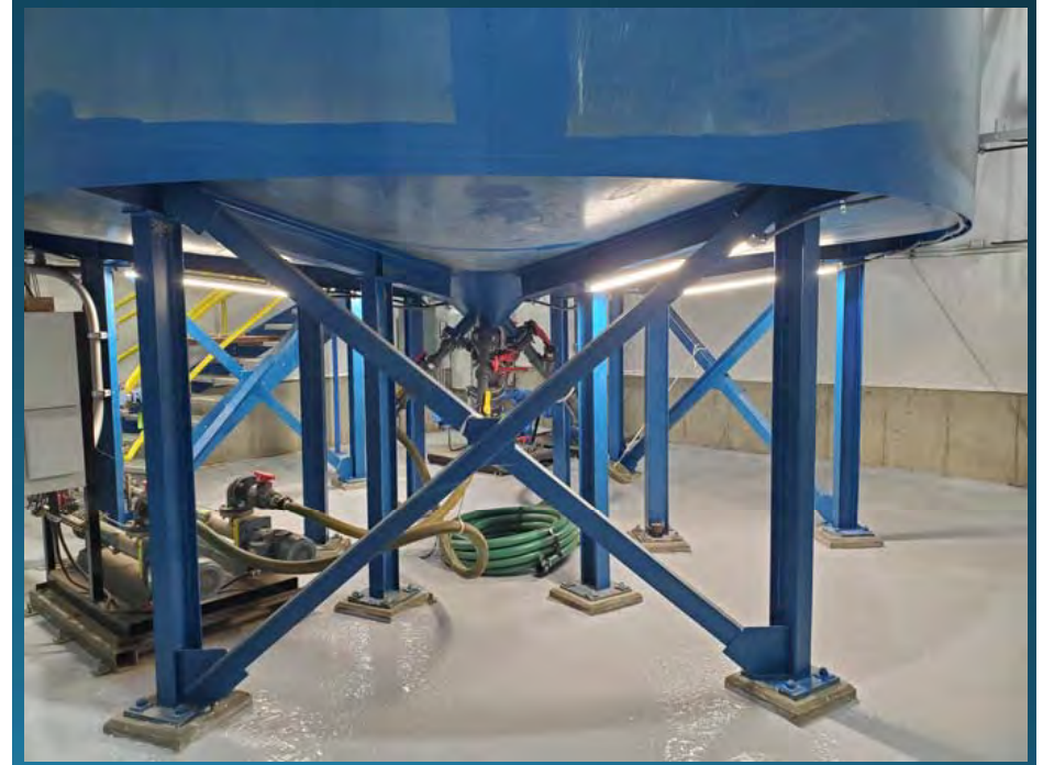
Sludge Recycle and Filter Press Feed Pump Skids
